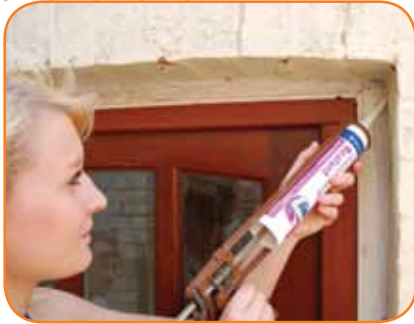
Figure 8.12 Sealing a door frame.
