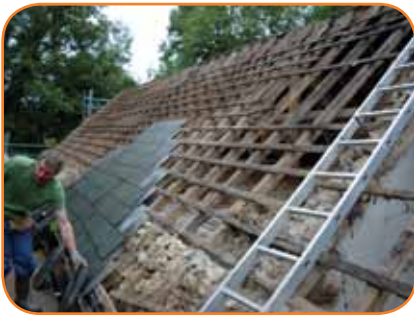
Figure 8.4 Slate being stripped for reuse. (Source: Nigel Griffiths)
